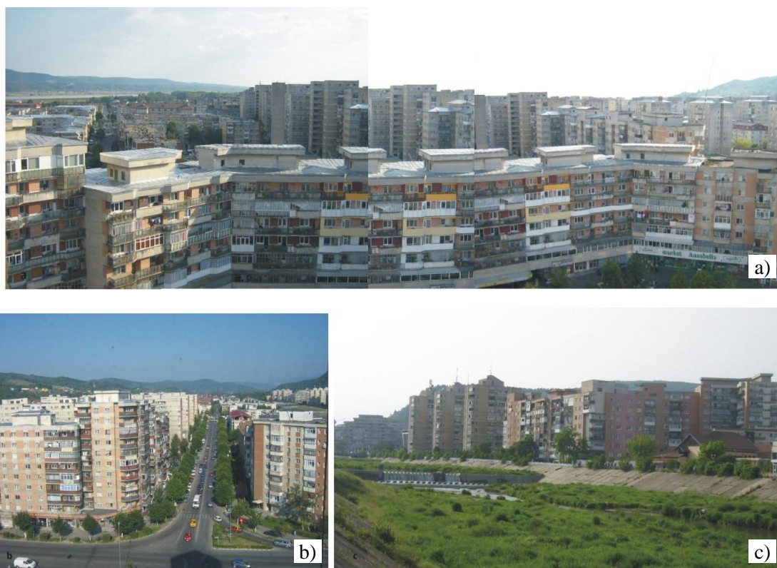
Figure 3. The Ostroveni – Râmnicu Vâlcea (South) great congregate-type habitat with a population of more than 50,000 inhabitants, built during the communist period for residential purposes and placed in the proximity of the southern industrial platform. a) south-eastern view; b) view towards the western part; c) the left front of Râmnicu (Cina Area)
